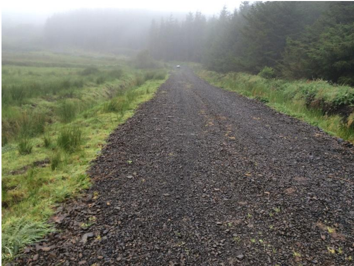
Plate 35: Route of proposed 33kV underground cabling along existing track further to south, looking NW.
