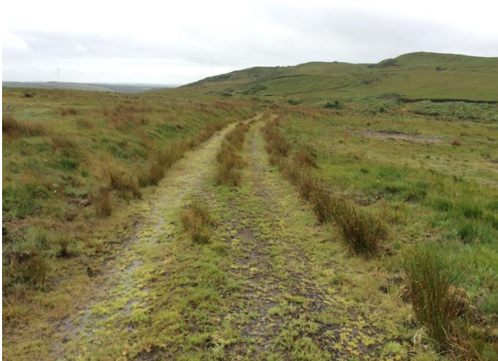
Plate 21: Road for upgrade, looking SW. Proposed borrow pit on right of photo, proposed temporary construction compound on left.
