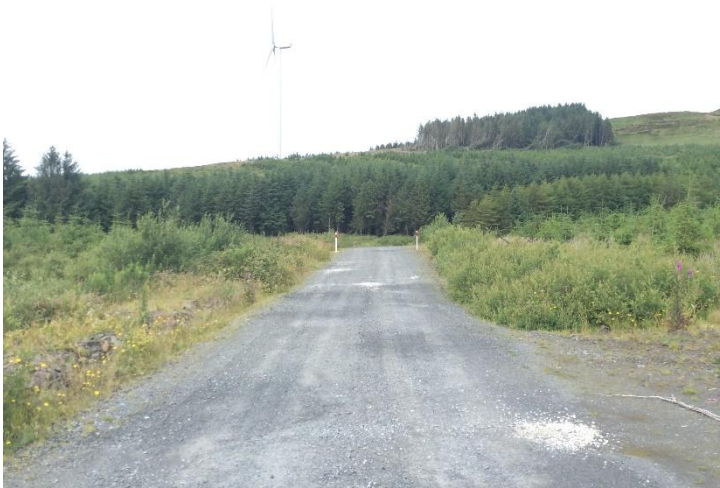
Plate 38: Route of proposed 33kV underground cabling along existing roads through the existing Slievecallan WF, looking N.
