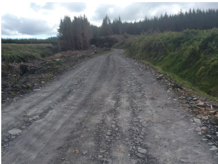
Plate 8: Existing road for upgrade SE of T1, looking SE.
