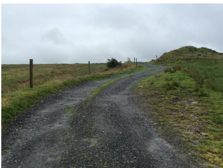
Plate 18: Existing road for upgrade north of T5, looking SE.
