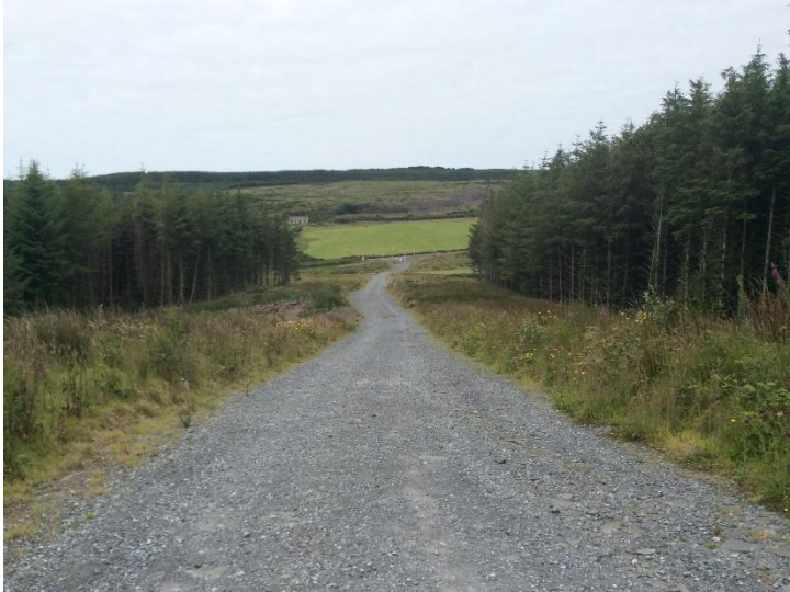
Plate 37: route of proposed 33kV underground cabling further to south, looking N. Protected Structure 637 background left.
